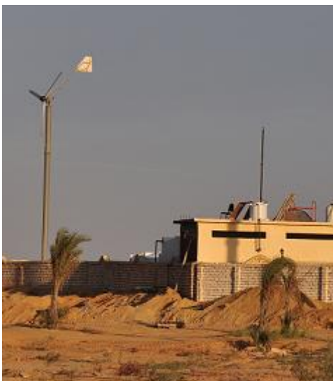
First Demo installation by Fortis with Montana 5 kW wind turbine
