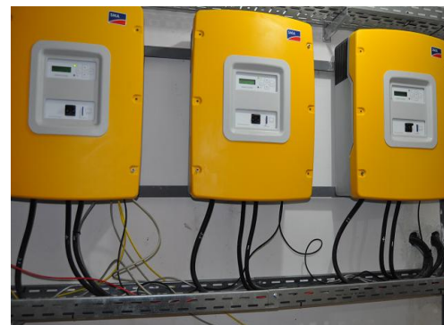
Sunny Islands battery Chargers /Inverters
