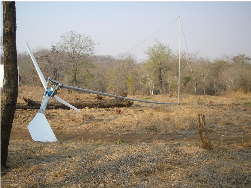
Wiring of 18 m guyed tower with Gine pole and Winch
